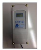
**Liquid Solution Temperature Control:** The liquid solution temperature control is an adjustable, microprocessor-based temperature control. This control receives temperature information from a thermistor located on the liquid solution supply line. A liquid crystal display continually indicates the liquid solution temperature. The control is mounted inside the chiller cabinet.
