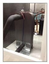
**Brazed Plate Heat Exchanger:** The heat exchanger (or evaporator) is of a brazed copper and stainless steel design. Refrigerant and liquid solution are channeled through the narrow openings between the plates and flow in opposite directions. The counter flow design and fluid turbulence ensures maximum heat exchange at minimal pressure drops.
